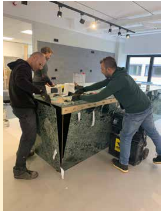
Constructing the new bar at Europalaan 93
